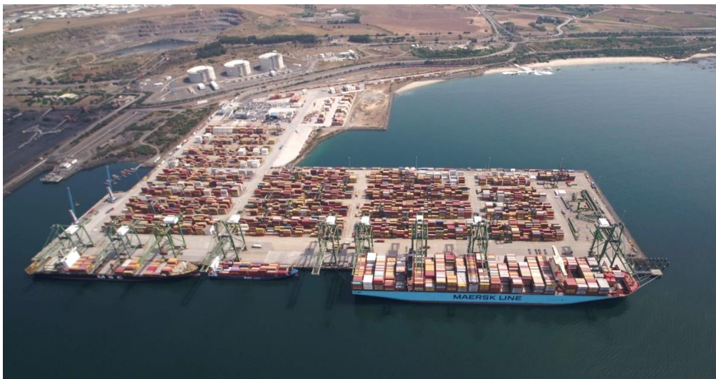
Figure 3.8 – Terminal XXI in the port of Sines
